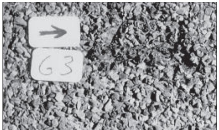
Photo A4. Close-up at fracture in Photo A3.
