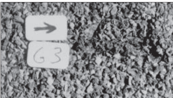
Photo 9. Close-up of Tab G-3, half-panel designation CO-FS-D-0 at 14 years 11 months weathering exposure. Note impact-caused fracture.
